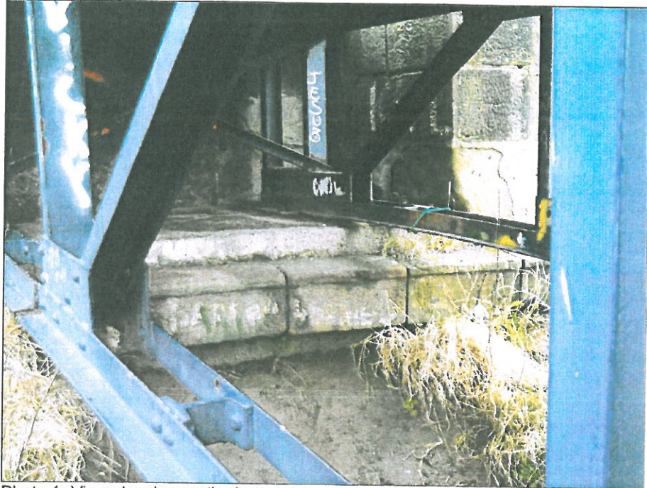
Photo 1: View showing north abutment bearing shelf
