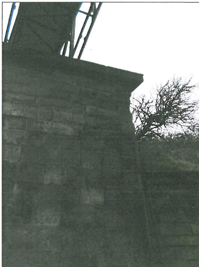
Photo 10: View of south pier- condition similar to north pier
