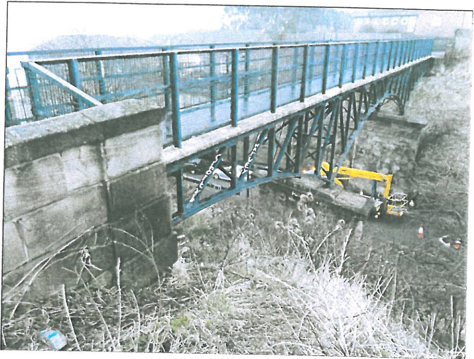
Photo 23: General view of the parapet
