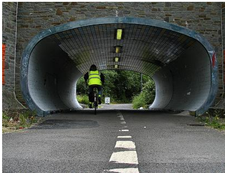
Photo 24 - Example of underbridge in Bristol
