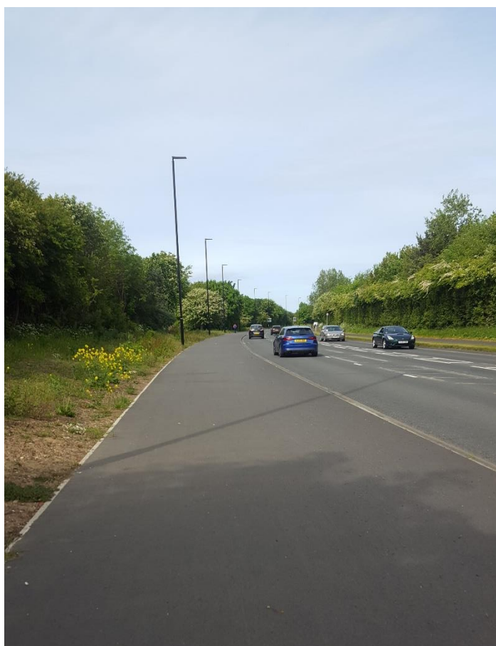
Photo 8 - Example of shared use route on Beach Road, North Tyneside
