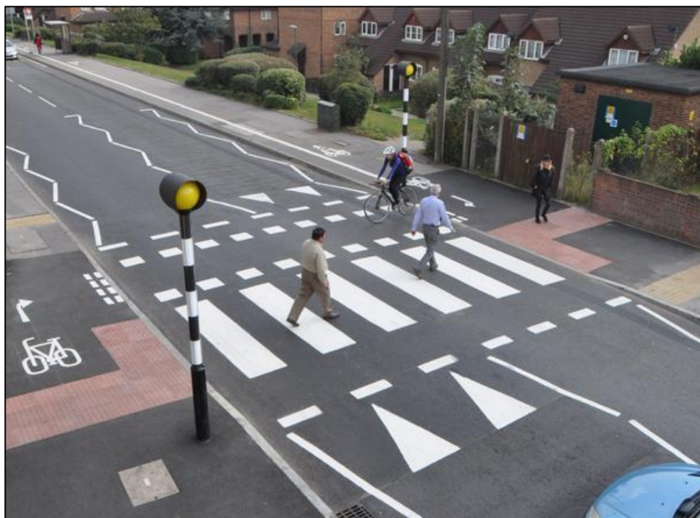
Photo 26 - Example of Parallel Crossing in Bexley, London
