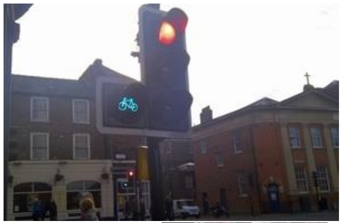
Photo 32 - Example of an early release traffic signals head
