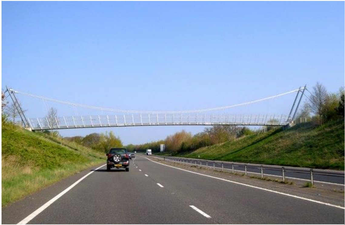
Photo 25 - Example of Footbridge over A5 near Nesscliffe Hill
