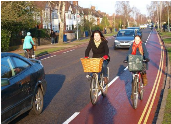
Photo 7 - Example of advisory cycle lane in Cambridge, these are represented by a dashed line
