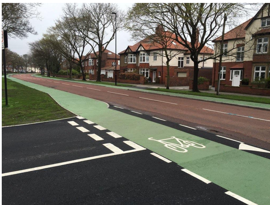
Photo 19 - Example of raised table at priority junction at The Broadway, Tynemouth
