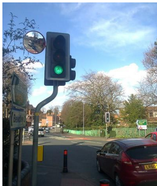
Photo 34 - Example of Trixi Mirror at signalised junction
