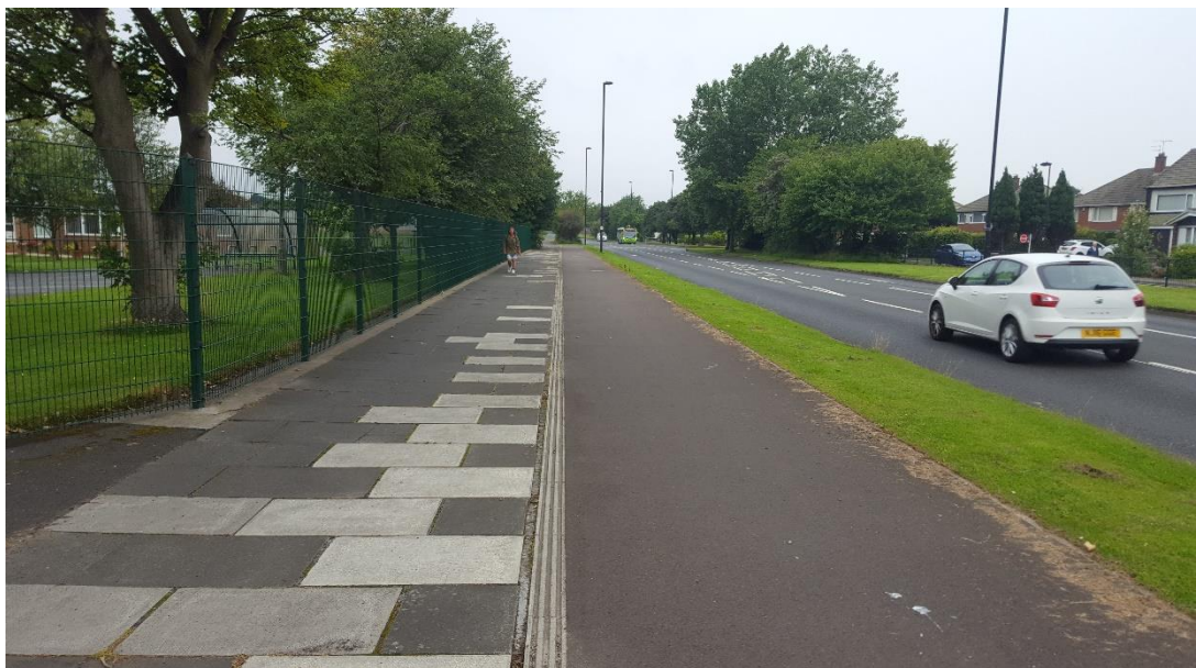
Photo 3 – Footway and Cycle Track on Beach Road, Tynemouth, clearly distinguished by surface treatment
