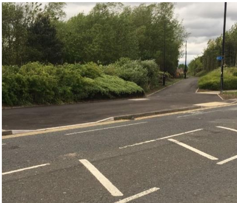
Photo 10 - Example of Transition Kerb into off road route at The Silverlink North, North Tyneside
