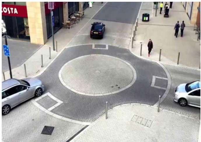
Photo 31 - Example of Informal Roundabout
