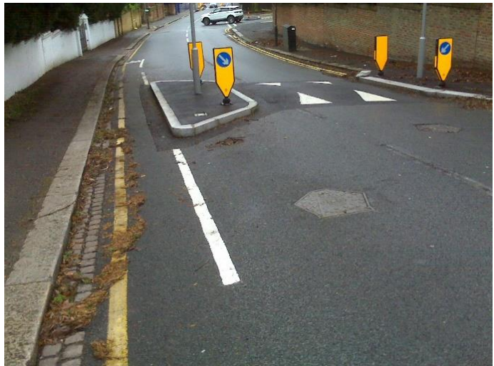
Photo 15 - Good example of cycle bypass at buildout for traffic calming
