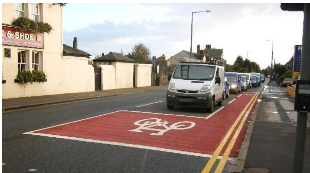
Photo 22 - Example of ASL with feeder lane
