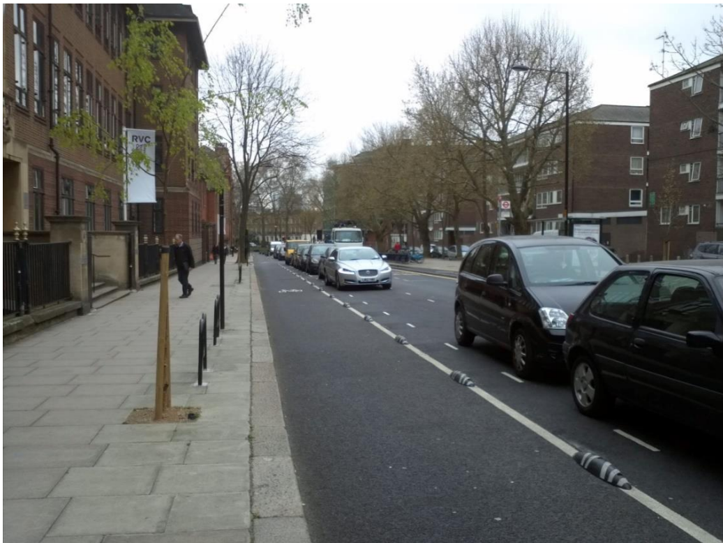
Photo 5 - Example of light segregation using armadillos (Pancras Road, London) – note inclusion of car door zone
