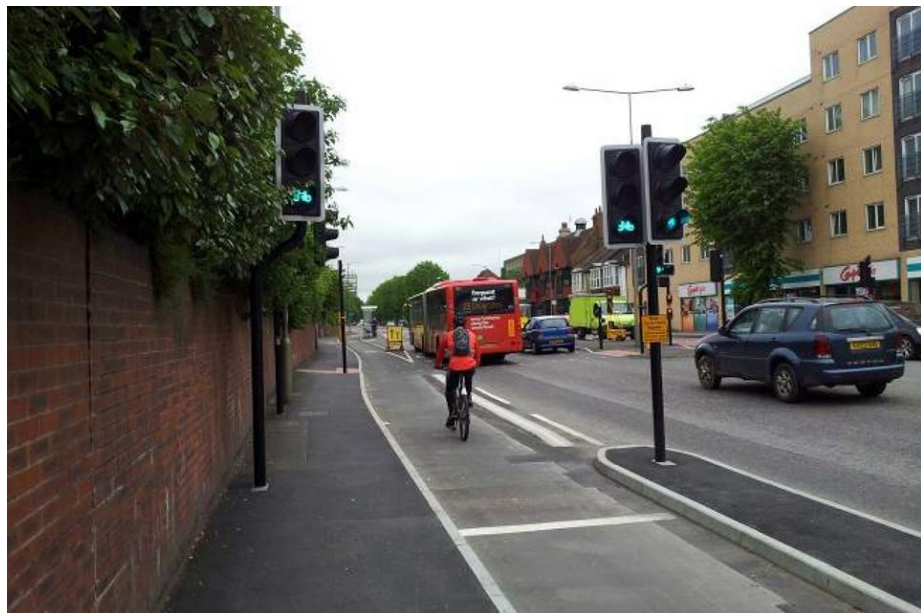
Photo 21 - Example of cycle bypass at signalised junction
