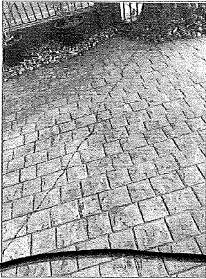
Photo - 82 Cracking to printed concrete parking area due to mature tree.
