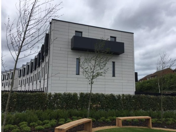
Modular Construction at Smiths Dock, North Shields
