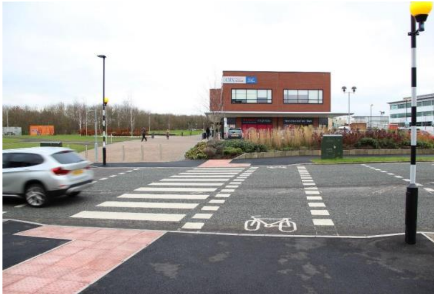
Image 12 - Parallel crossing in Cobalt, North Tyneside
