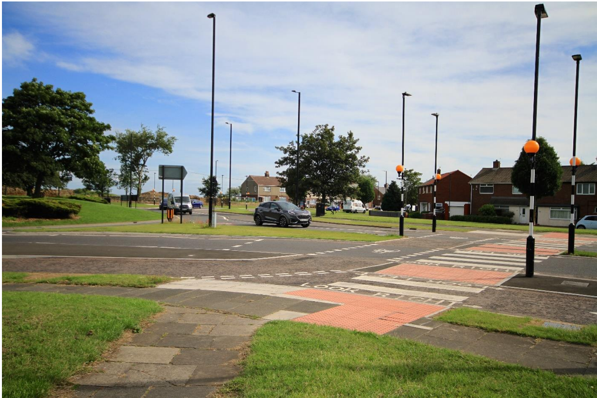
Image 11 – Roundabout with protected space for cycling in North Shields, North Tyneside
